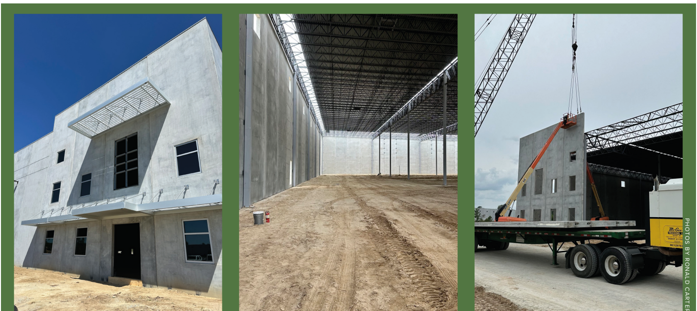
The 101,500 sq ft building in the Georgetown County Business Center in Andrews was completed in September. Empty precast concrete-walled boxes with high ceilings and no floors allow for a variety of manufacturing uses. This flexible, open design will make it easier for manufacturers to move in and begin production.
